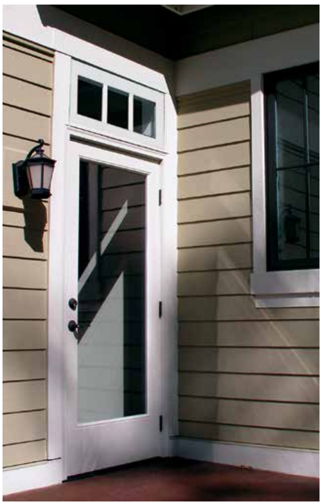
SF20F door with Bright paint.
